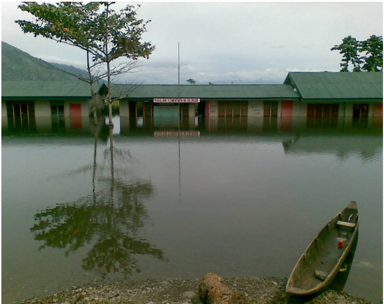
Figure 14: An elementary School in Underwater during a flood (MAO)
