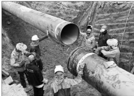
Building the Chad-Cameroon pipeline
