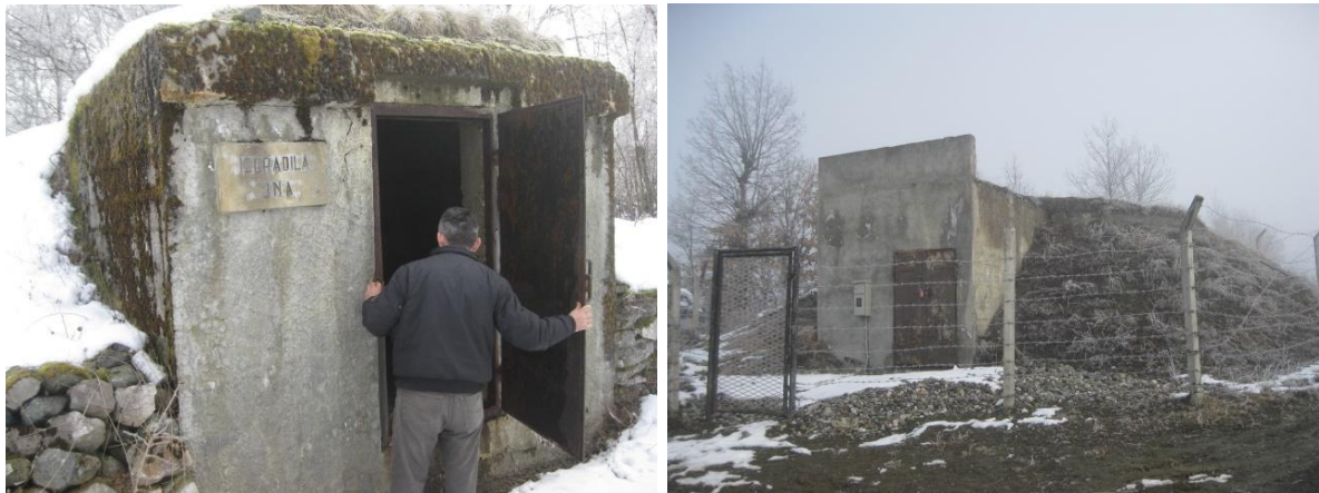
Figure 4: Reservoirs Zova I (V=50 m 3 ) and Begova voda (V=250 m 3 )
